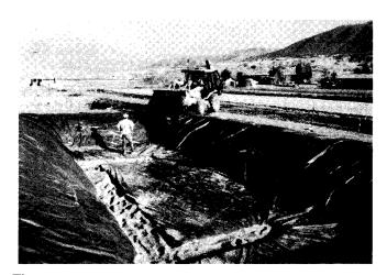
Figure 2-Smallest pond during construction, showing subsurface drain system and 30-mil plastic liner.
