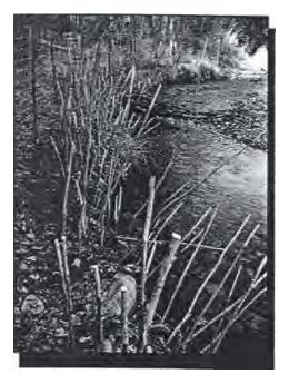
Figure 1—Cuttings were planted to stabilize an eroding creek bank.— Kristi DuBois photo
